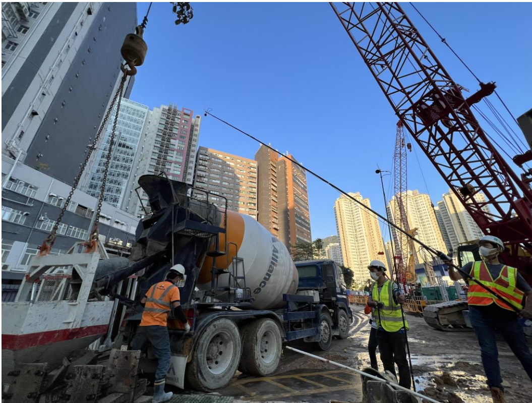
Photo C2. Measurement Photo for Concrete Discharge Mode
